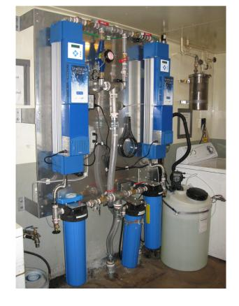
vessels or fleets, and more specifically, the application of an Ultra Violet System as part of a system to ensure the safety of a vessel's potable water supply." To that end the consistent positive results have proven that the application of the Upstream® Ultra Violet light by UV Pure® was and remains the right choice.
