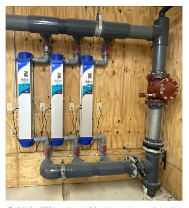
Each Hallett 1000 is equipped with four integrated sensors that continually monitor UV transmittance and UV intensity. This unique feature eliminates the need for an external UV sensor and can boost capital cost savings by as much as \$15,000.
